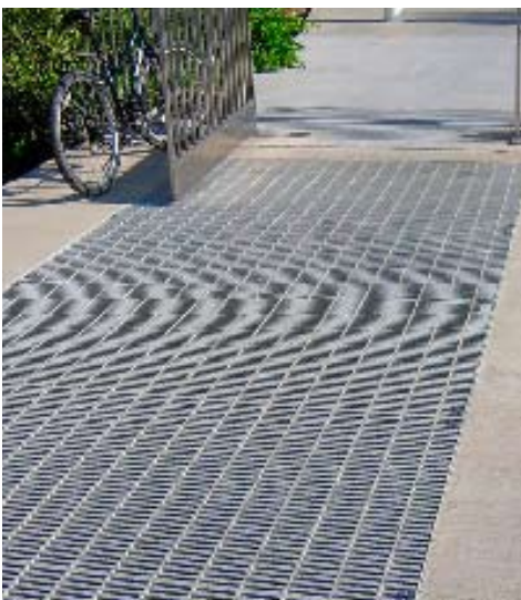
Fibergrate grating used to cover a trench walkway allowing for drainage and safe pedestrian passage
