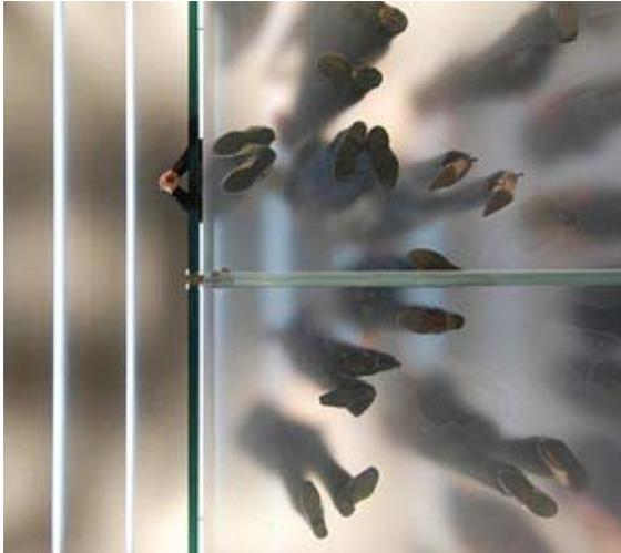
Man leans over balustrade of laminated safety glass. Apple Store staircase and balustrade, Regent Street, London (UK), with illuminated laminated glass roof by Carpenter-Lowings (2004).
